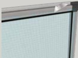
Then using the concave end of the spline roller, push down and roll forwards whilst keeping the mesh pulled straight with a gentle tension, but not too tight.
